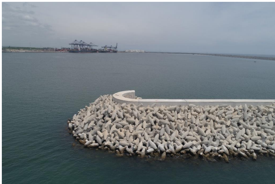
Image G. View from the southern section of the west breakwater to the port's expansion terminals.
